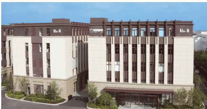
STAUFF China headquarter | Songjiang District, Shanghai
